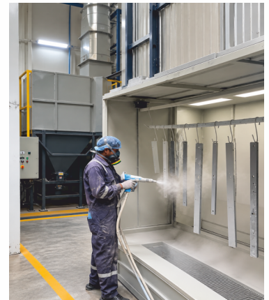
Powder Coating Plant
